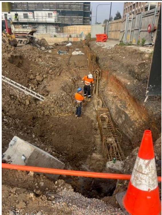
Photos 1 & 2: Construction of capping beams and basement excavation on southern side of Conferta Avenue
