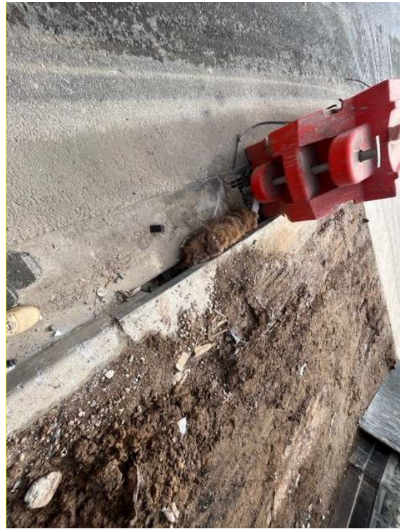
Photos 19&20: Disturbed soil was spilling into the gutter on Conferta Road. The controls around the stormwater drain in this location were inadequate, posing a risk of sediment entry.
