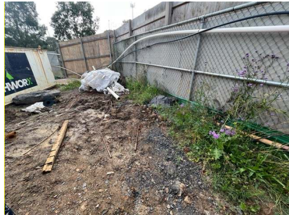
Photos 9-12: Sediment fencing was in poor condition along the southern boundary of the site. Housekeeping improvements were also required along the boundary.
