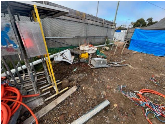
Photos 9-12: Sediment fencing was in poor condition along the southern boundary of the site. Housekeeping improvements were also required along the boundary.
