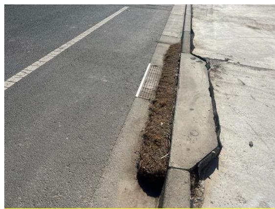
**Photo 19:** Coir logs and geofabric controls at stormwater inlets on Conferta Ave
