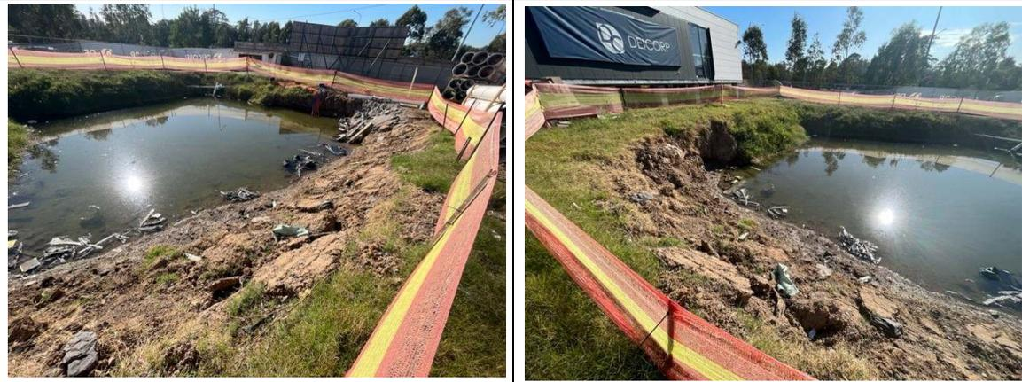
**Photos 7 & 8:** Sediment basin, SE corner of Site 2. Rubbish recommended for removal, as well stabilisation and seeding of the disturbed batter.
