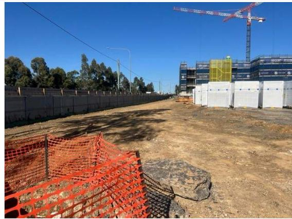
**Photo 13:** Site 2 – Additional stabilisation of ground surface in the SE corner recommended
