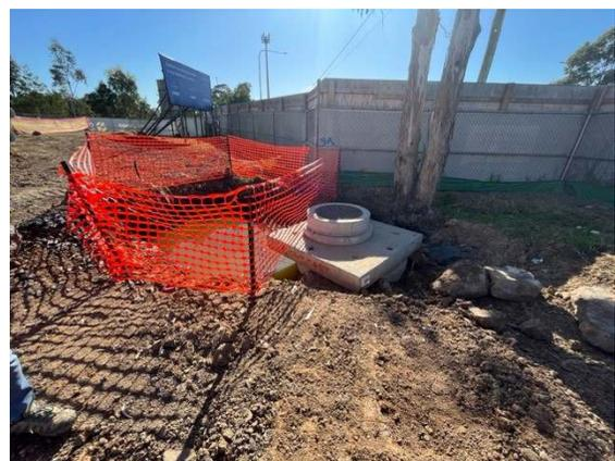
**Photos 23 & 24:** Tree damage from sewer installation in SE corner of Site 2. Deicorp advised tree does not require retention and would be removed prior to Stage 3 works commencing
