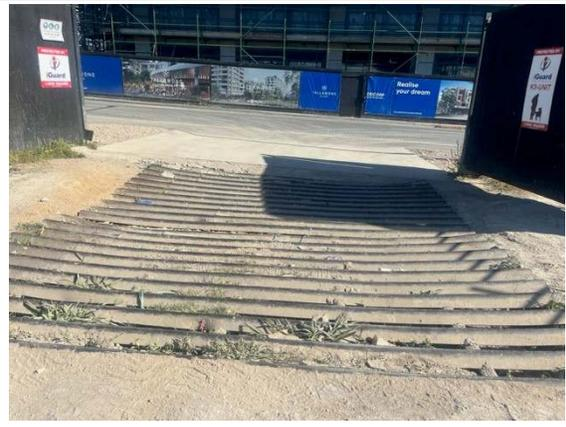
**Photo 14:** Shaker grid at lower Site 2 access
