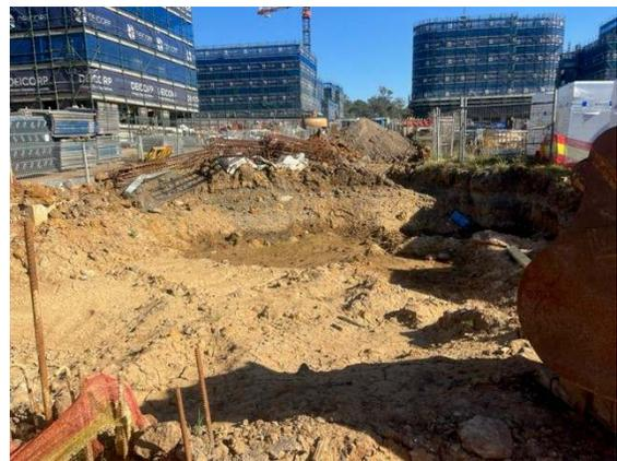
**Photo 22:** Site 2 – Stockpile area – recommended for dust suppression and cover at end of each day
