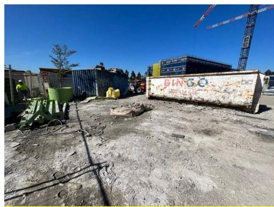
**Photo 20:** Waste storage and concrete washout area
